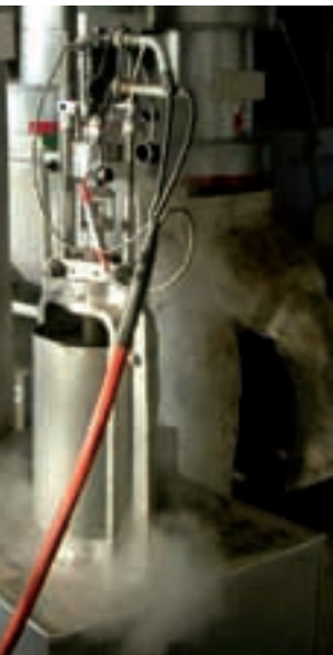
Hydraulic test equipment in place, ready for testing the safety valve
