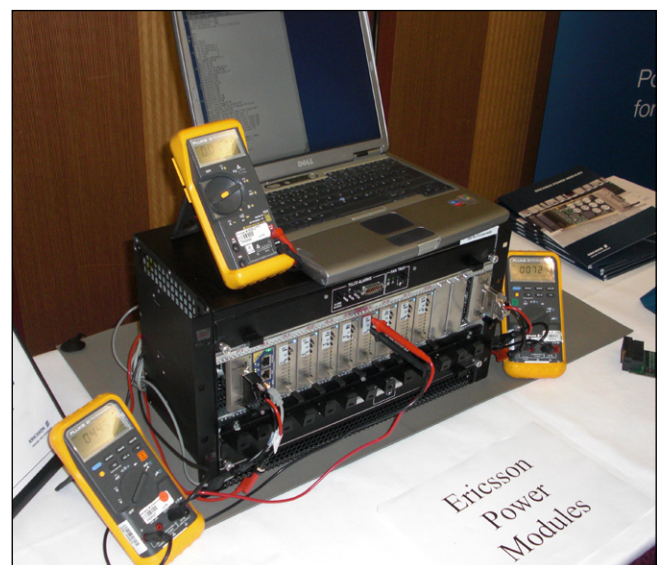
Figure 9 - Photo of MicroTCA system with test equipment for measuring current and voltage levels
