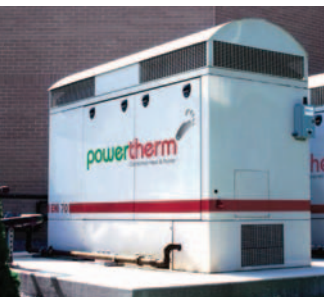
Scorpion Power Systems' CHP offering is based on a natural gas engine-driven generator
