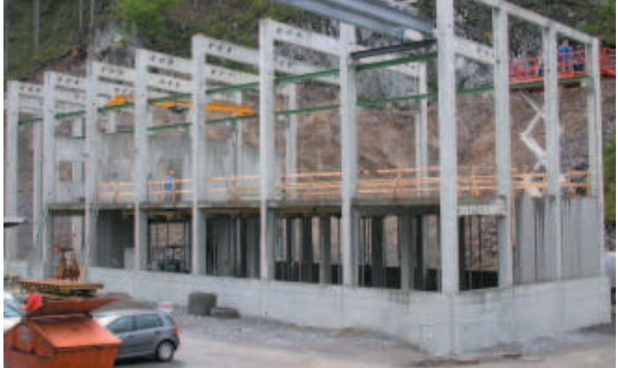
Ceratizit's tungsten carbide recycling plant goes up in Austria. The company is piloting a customer tip recycling programme in Germany and will roll it out in the UK soon
