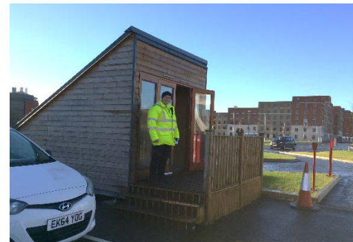
It now provides a home for the Security staff on the Bay Campus
