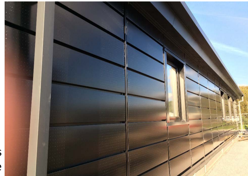
New Coretinium wall panels
