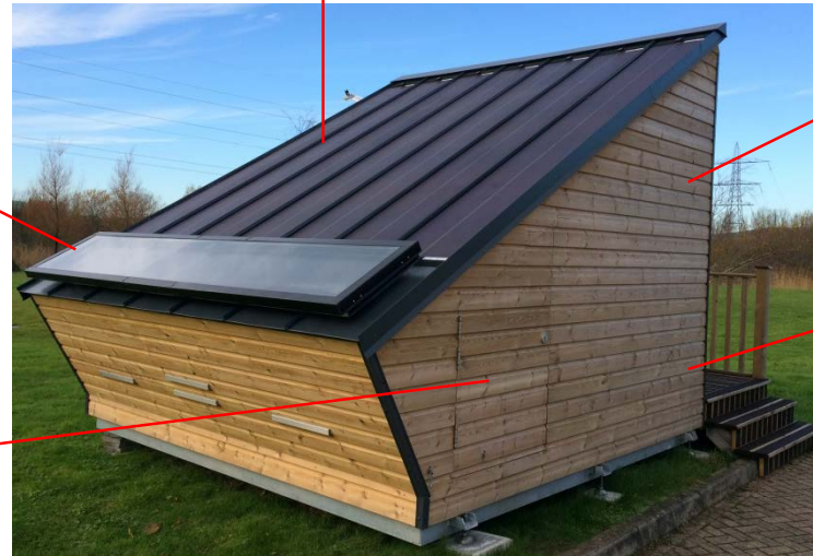
Building Integrated Photovoltaics (BIPV) - electricity
