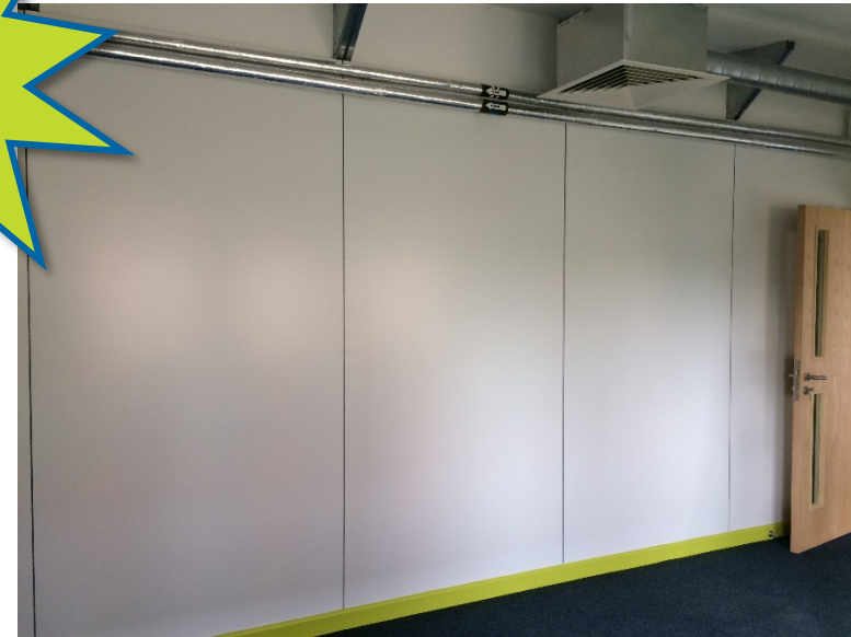
New Coretinium wall panels
