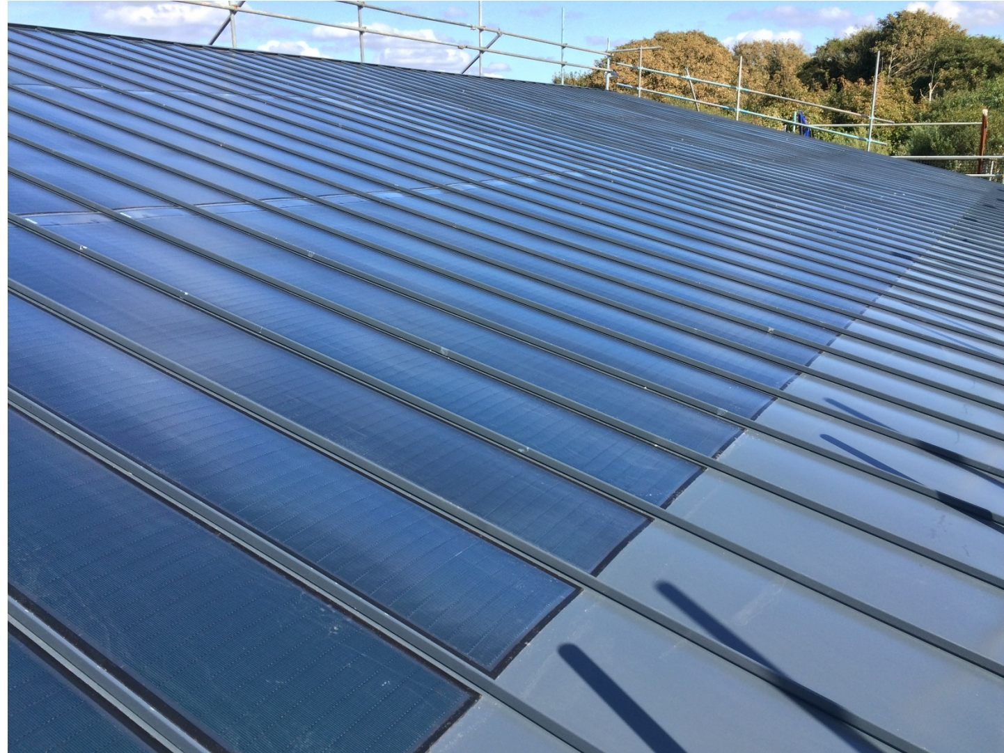
First BIPV Co roof in the UK – generating approx. 17kWp of electricity
