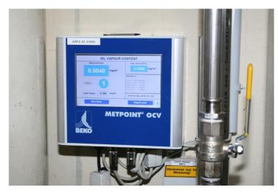
Besides the great plus for the process safety regarding the compressed-air supply, project engineer Harald Kunkler reckons with another positive effect of the new residual oil monitoring: "Until today, there was always an uncertainty between the sample checks concerning the degree of saturation of our oil vapour adsorbers, and therefore concerning our process safety. With the METPOINT OCV devices, we will be able to detect.
