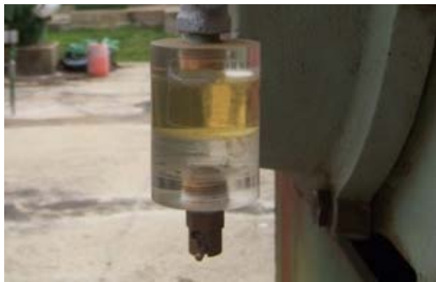
Figure 4. An oil sight glass (bottom sediment and water bowl) installed on a drain is a great indicator of problems such as water ingress or degraded oil.
